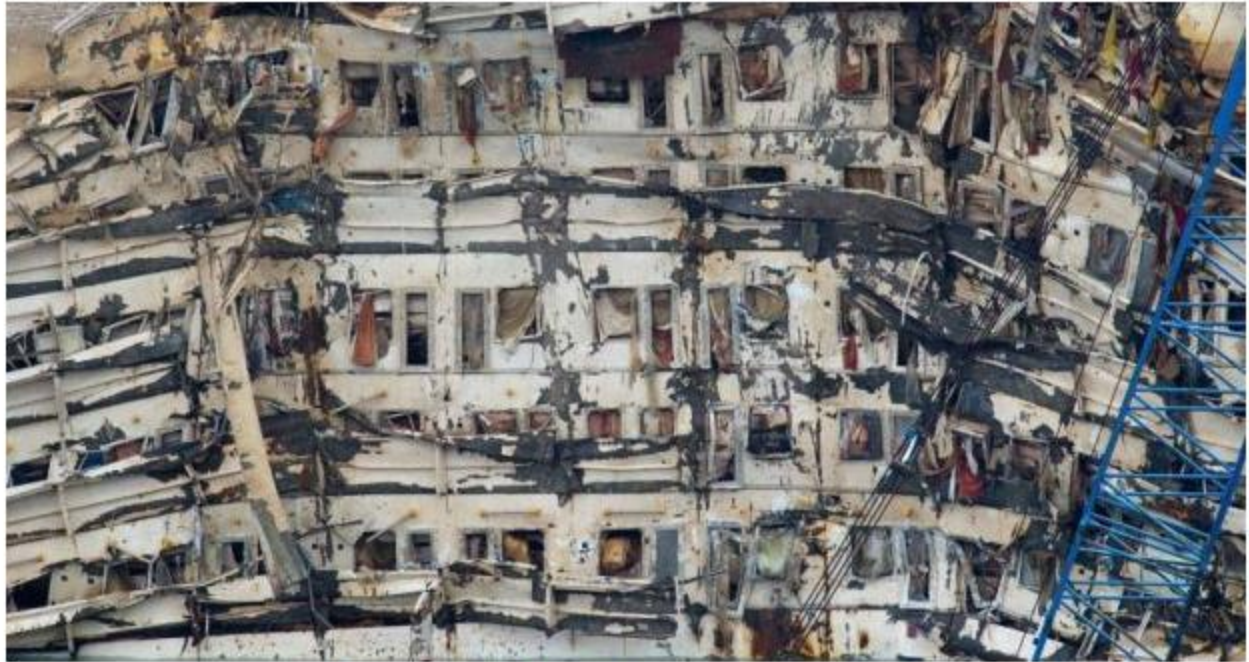
Costa Concordia upright after 19-hour operation
